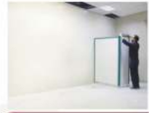
8 Adjusting & leveling from the other side
