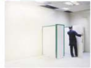
16 Mounting of door leaf for the second unit
