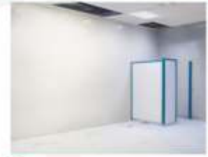
12 The first unit of lavatories is ready for door leaf mounting
