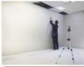
5 Marking the final elevation
