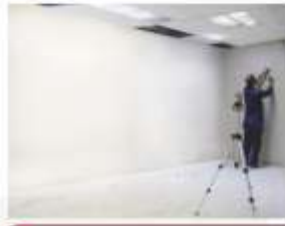
6 Marking the final elevation in different points
