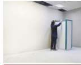
7 Adjusting & leveling the first panel
