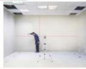
3 Specifying floor elevation levels by laser device
